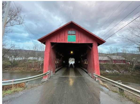
West Portal Looking East
