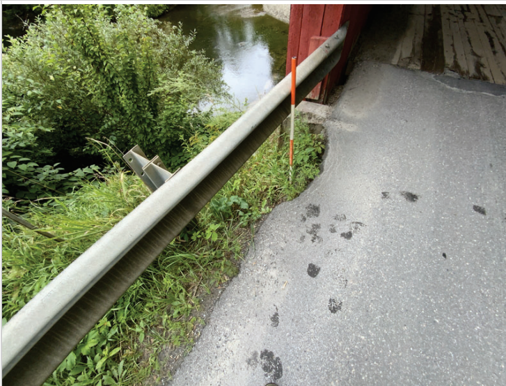
Upstream abutment 1 shoulder area
