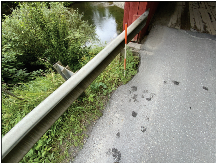
Upstream abutment 1 shoulder area
