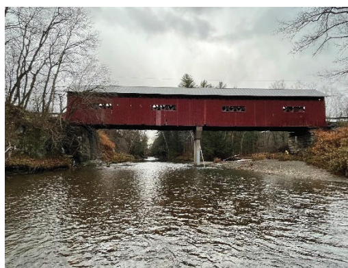
Downstream Elevation Looking South
