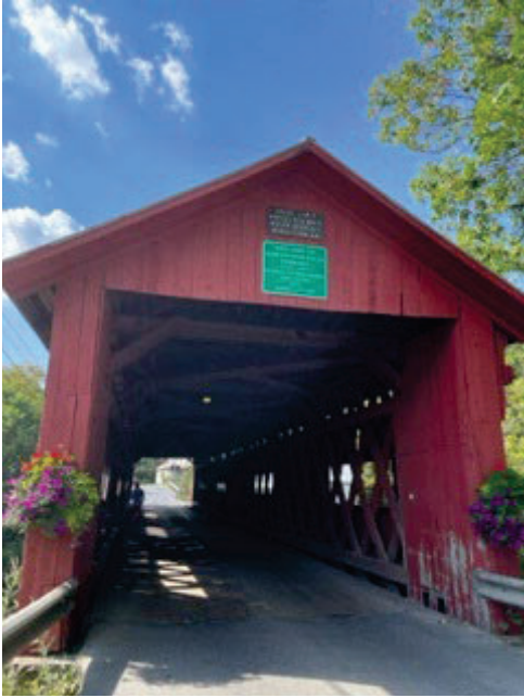
Bridge 10, taken on 9/6/2023
