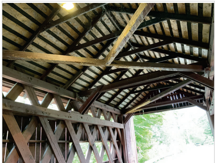
Lateral cross bracing
