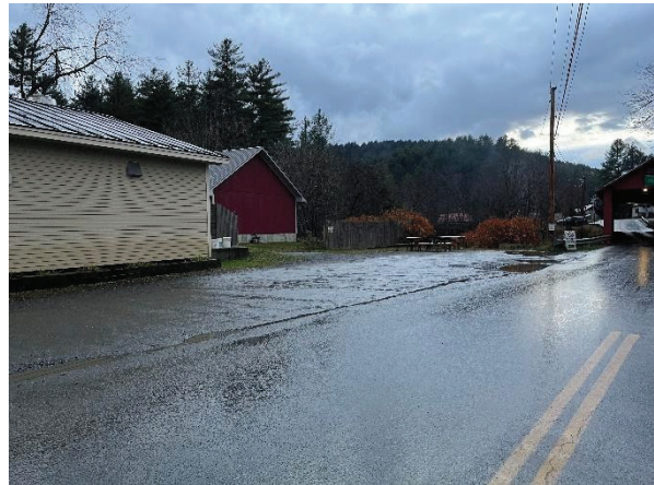
Commercial Drive at South Approach
