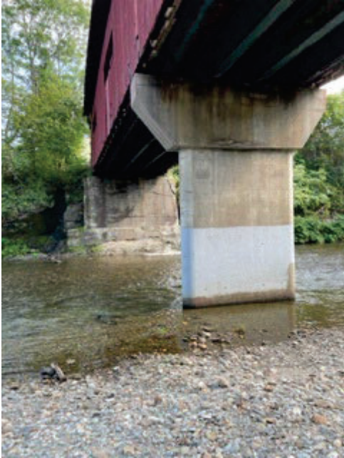
The underside of bridge 11. Taken 9/6/2023
