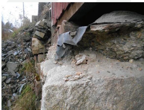
West Abutment Beam Seat
