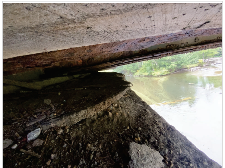
Abutment 1 beam ends
